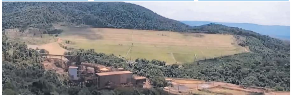
Disaster: The Brumadinho dam before, above, and moments after its wall collapsed.
